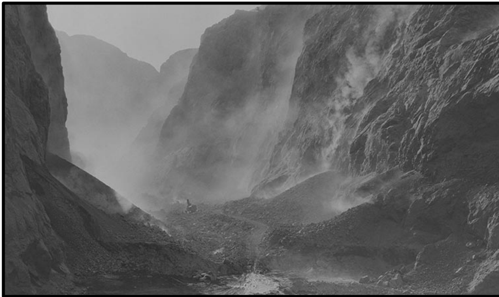
Figure 8: Construction at the Hoover Dam site, circa 1934 (NPS LAKE 2017).
