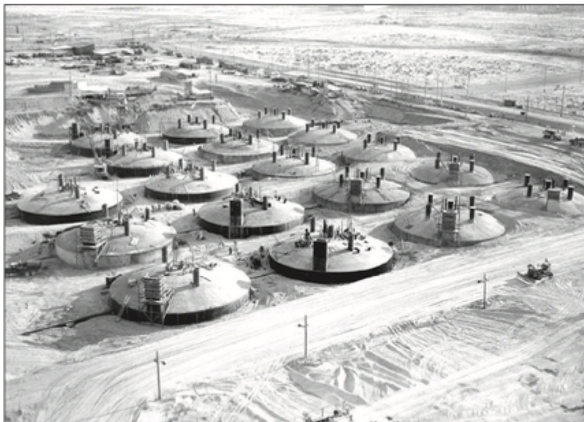
Figure 3: Hanford site tank farm 241-TX being backfilled [22].
