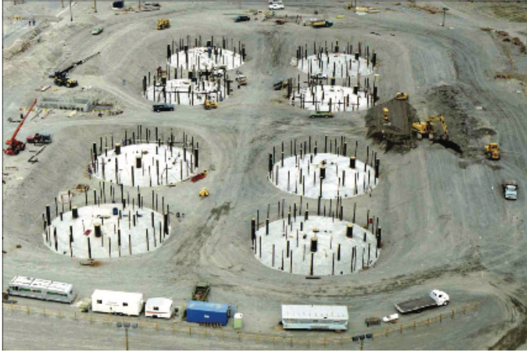
Figure 5: Hanford Site DST farm 241-AP nearing backfill completion [22].
