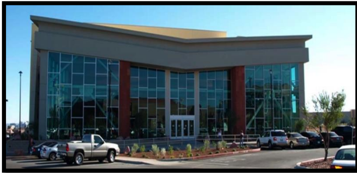
Figure 6: Exterior View of Library
